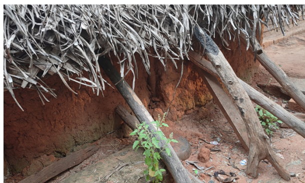
Figure 8. Most CIHs (climate impacted households) has walls and rooves that were weak and vulnerable to cyclones and heavy rains.
